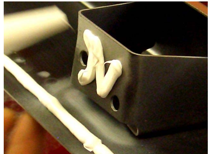
FLOOR EXTENSION REINFORCEMENT
